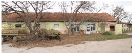
Figure 3: The old building in Petrich before the restoration
