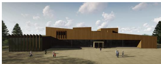
Figure 4: The old building in Petrich after the restoration
